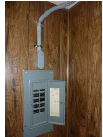
Branch off Building Main Panel for Sub Panel in Press Room
