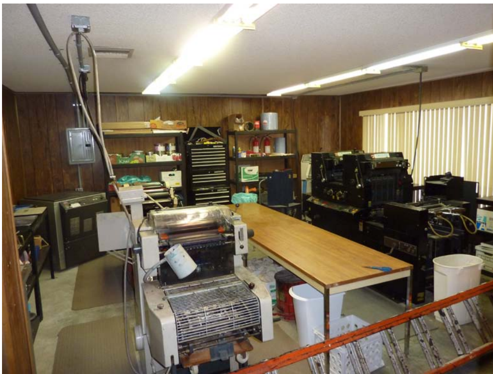
Ceiling plugs in Press room from new 90 AMP Sub Panel Three 220 volt and two 120 volt designated outlets
