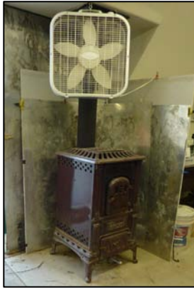
A Plugger's forced air heating system
