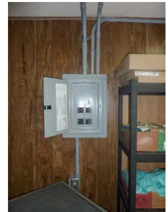
90 AMP Sub Panel in Press Room
