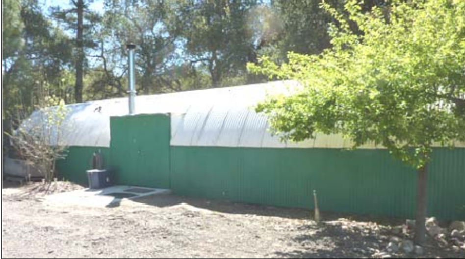
860 Square Foot Remodeled Quonset hut for Christian Evangelism Printing
